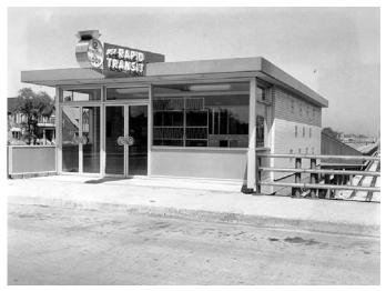
panels alternated with ventilation louvers. This glass month before entering service, was typical of the 1958 Congress was later removed, effectively making the ramps open Line station. Note the neon entrance sign and signature door handles.
